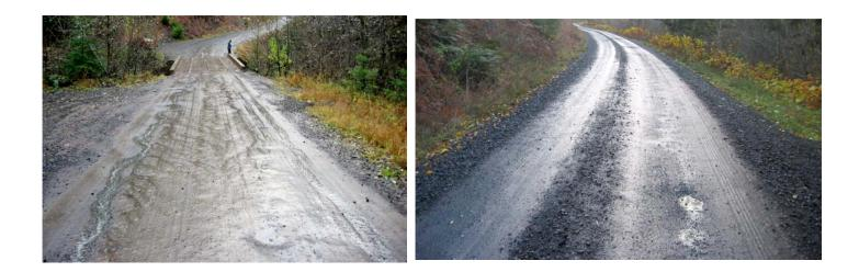
**Photo 1a & b.** Two roads in the Oregon Coast Range that had been surfaced with rock and gravel about 3 months prior to the time of photos. The travelways had primarily reverted to a native surface condition that is actively eroding, including that in concentrated runoff in ruts in the native surface of the roads, resulting in high levels of sediment delivered to nearby streams.
